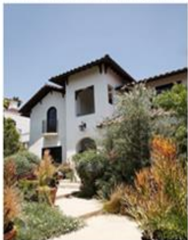
Architect (obby Rees restored the 1920s house to its original Spanish-inspired style.
